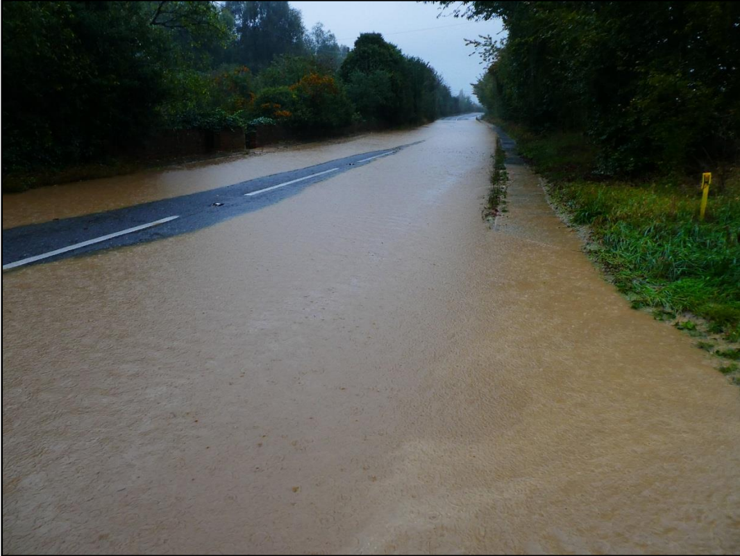
Image 3. Parham highway flooding
