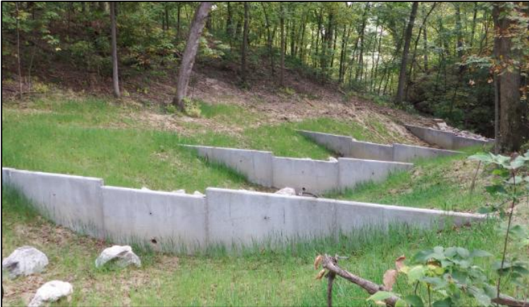
Photo 13: Concrete Checks Dams Example (Bur Oak Land Trust)
