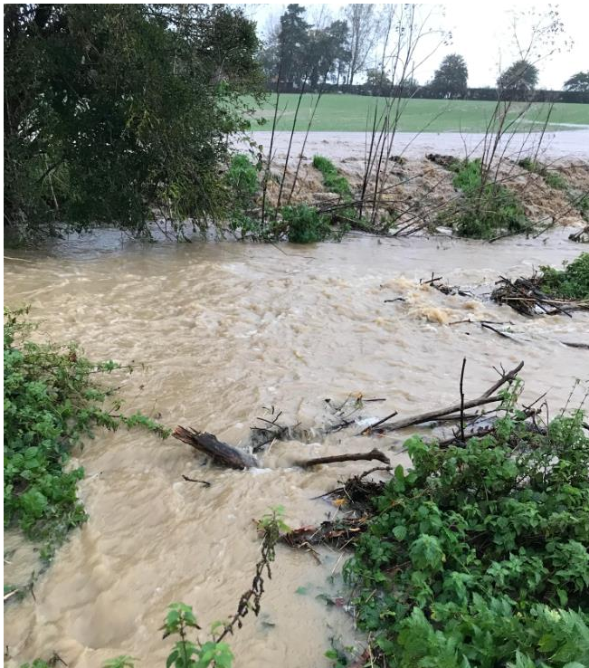
Culvert opposite Garnetts garden centre over flowing on to B1116 Photo taken facing sSouth West W3W ///various.upwardly.diamonds
