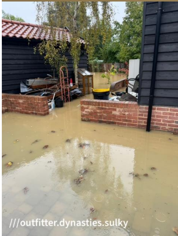
Photo taken facing North water levels were up to 700mm deep here at 6pm
