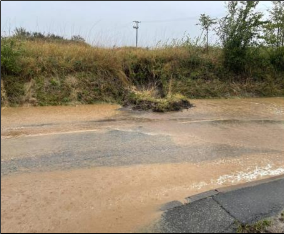
Photo 9: Bank on western side of 'The Street' opposite Thatched Cottage failure due to saturation.
