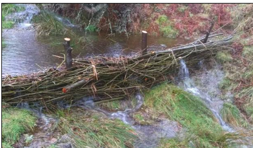
Photo 12: Leaky dam constructed across watercourse in Dartmoor Headwater Natural Flood Management Project (Dartmoor National Park).
